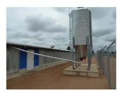
Enclose all transfer points along the feed storage and distribution system to minimize emissions from the feed and feed transfer.
