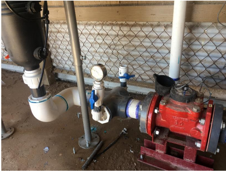
Figure 1. New filter system and repaired water-meter.
