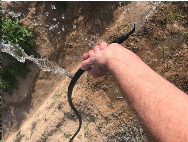
Figure 4. Damage due to equipment or possibly vandalism
