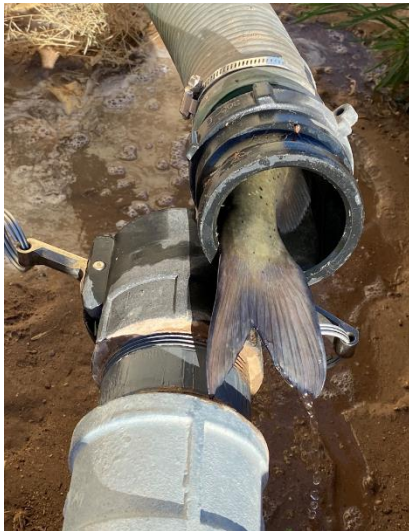
Figure 1. Fish caught in irrigation pipe. This fish could not enter the irrigation pump because of a screen in the line but needed to be removed by hand.
