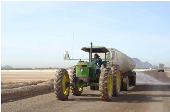
Watering is a BMP in the non-cropland category. Applying water from a truck, tractor or other portable sprayer to unpaved roadways and equipment yards, will help reduce PM10. Watering the soil surface tends to compact the soil so that it is not dispersed into the air.
