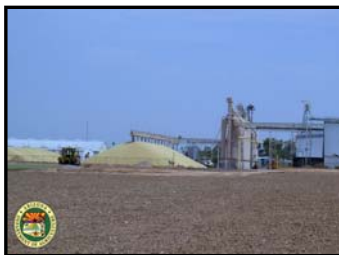
Grain facility - ADA-PSD
