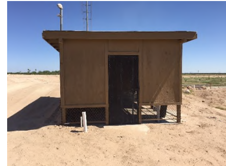
Figure 2. Pumphouse at the north end of Block 6.
