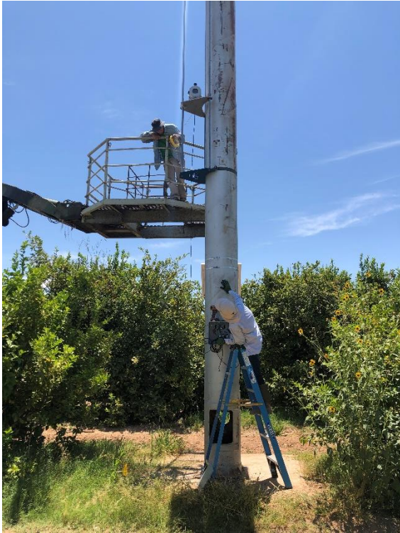
Figure 3. Installation of instruments and data loggers to wind machine towers
