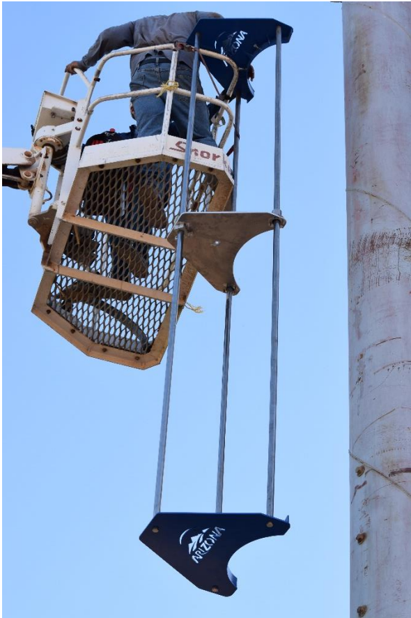
Figure 1. Installation of an adjustable mechanism platform
