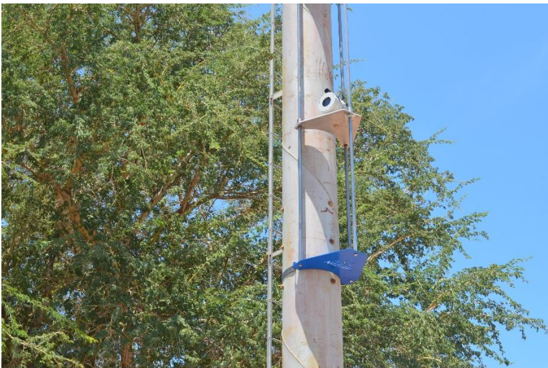
Figure 4. Transmitter affixed to tower
